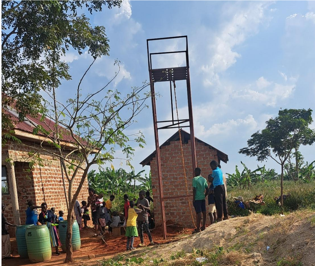
Stand for 1000 litre water tank in place to be filled from new borehole
